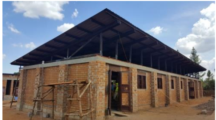
Week 19 Progress Roof structure erected
