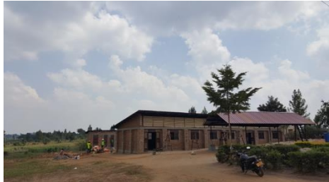
Week 20 Progress EcoSan, main building and shelter all structurally complete
